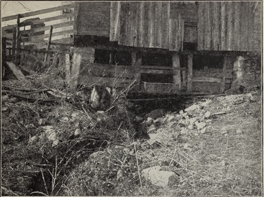
FIG. 1.—Insanitary conditions at small local slaughterhouse. Note the exposed drainage. Hogs are often fed on offal under such abattoirs, and rats and other animals have free access, thus favoring the spread of disease.
